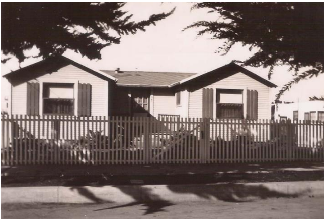
Tent City cottages in Imperial Beach represent how reuse can generate new development in a sustainable way (South Bay Historical Society).
