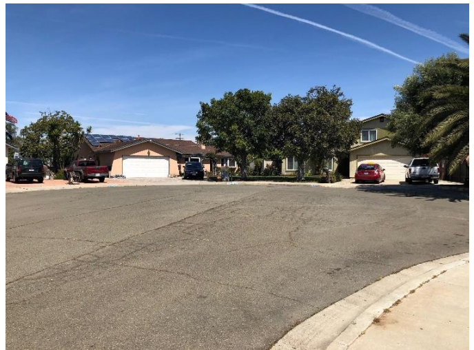
Dead-ends and cul-de-sacs create barriers to an open and connected community. (Photos: Tim Briggs).
