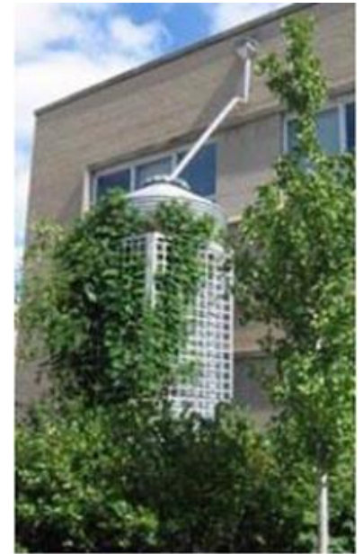
Bioswale (top) and rainwater harvesting (bottom) are examples of green infrastructure.
