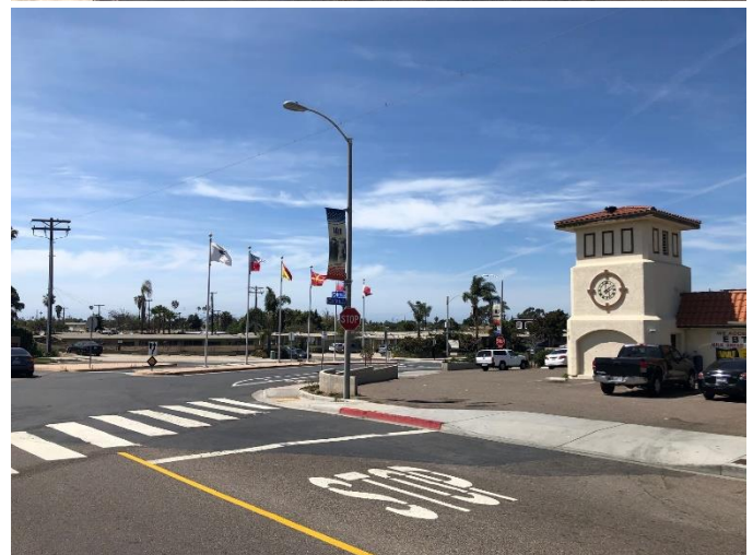
Existing conditions at future walkable centers at Seacoast Village (top), Miracle District (middle), and Aviation Center (bottom). (Photos: Tim Briggs)
