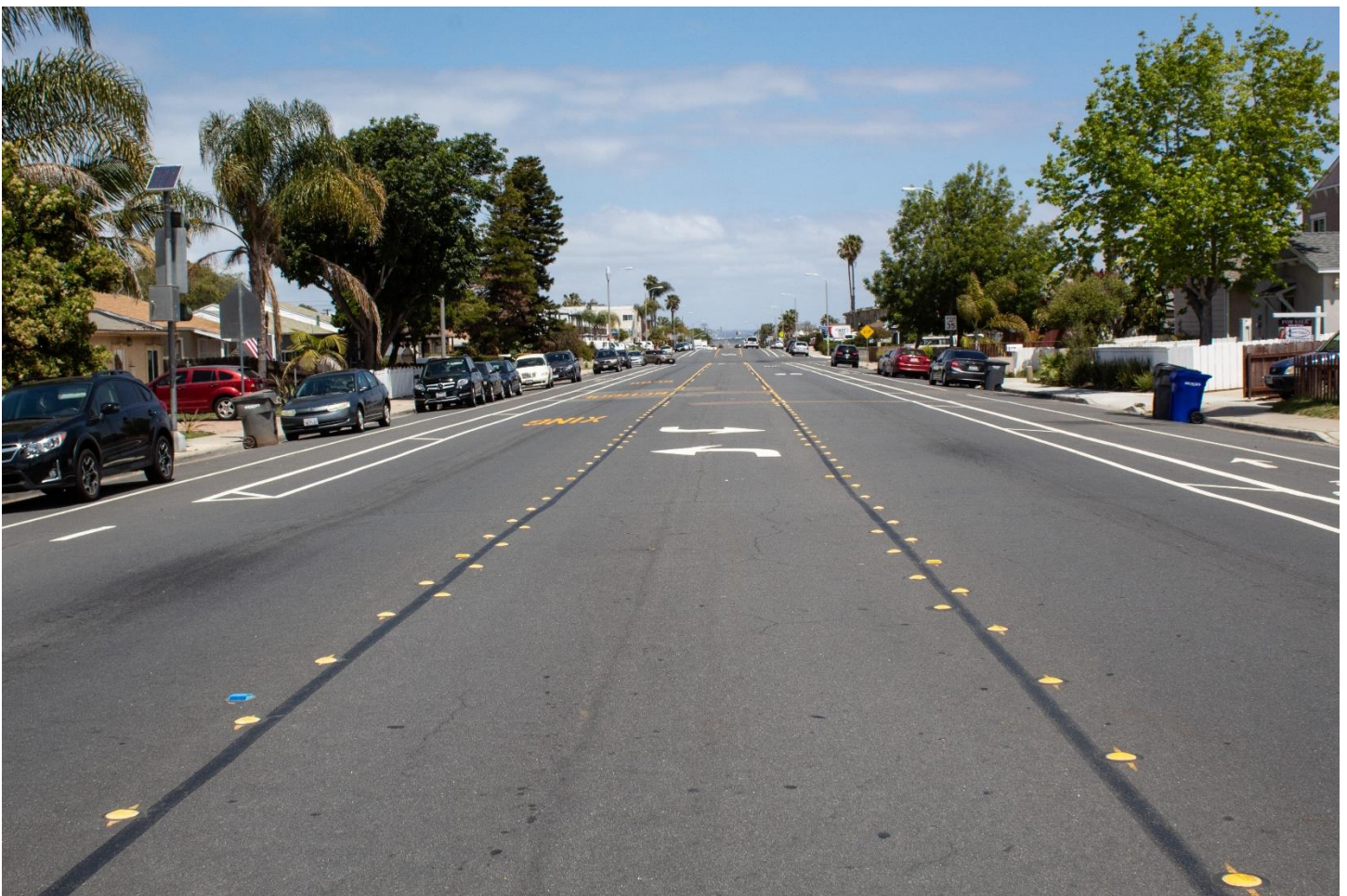
Looking north on 13 th Street. Photo: Brittany Cabeje
