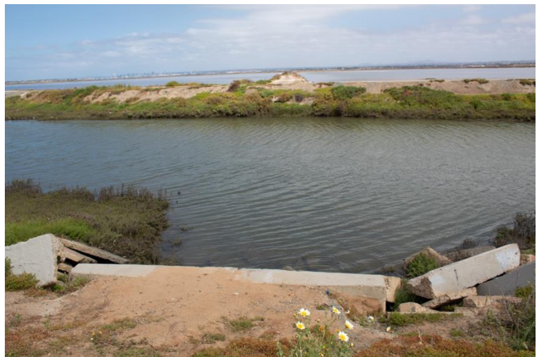
Storm drain at Bayfront Park. Photo: Brittany Cabeje.
