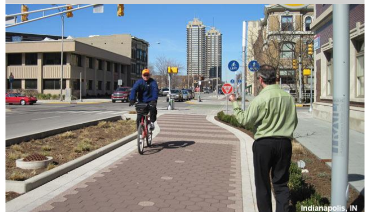
(from top) Corridor enhancements include: multiway boulevards, t-intersections at frontage streets, gateway curb extensions at those intersections, and separated cycle tracks (Photos: NACTO).
