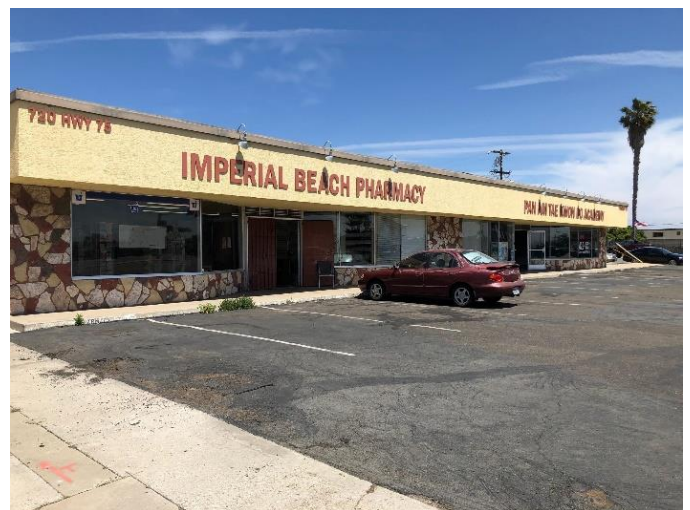
Single family homes and shopping strips are characteristic of the sprawling development pattern in Imperial Beach. (Photos: Tim Briggs)
