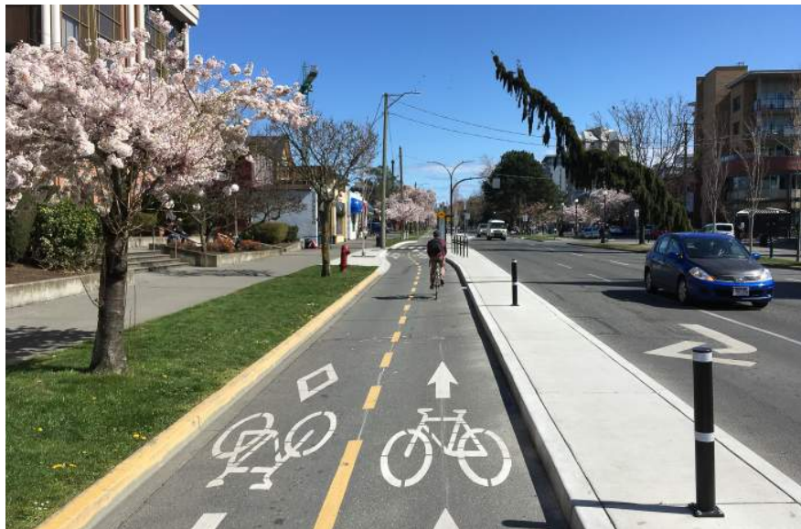
Top: Two-way facility Washington D.C. & Bottom: Two-way facility Victoria, Canada
