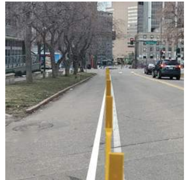
Eighteen-inch painted buffer with plastic delineators
