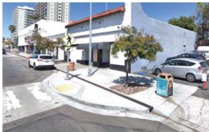
Curb Ramp with Trench Drain: Park Boulevard and Essex Street, San Diego, CA
