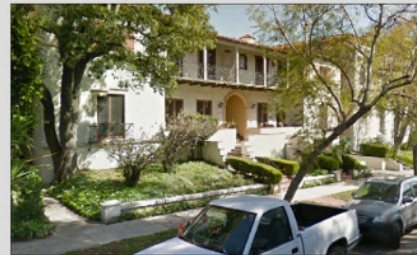
Above: Courtyard building with stoop frontage leading to central entry to courtyard through zaguan in center of photo. Street facing units are entered from the street and from the courtyard.
