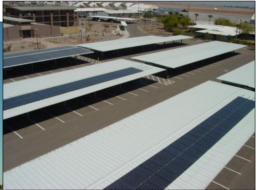
Carport Photovoltaic System
