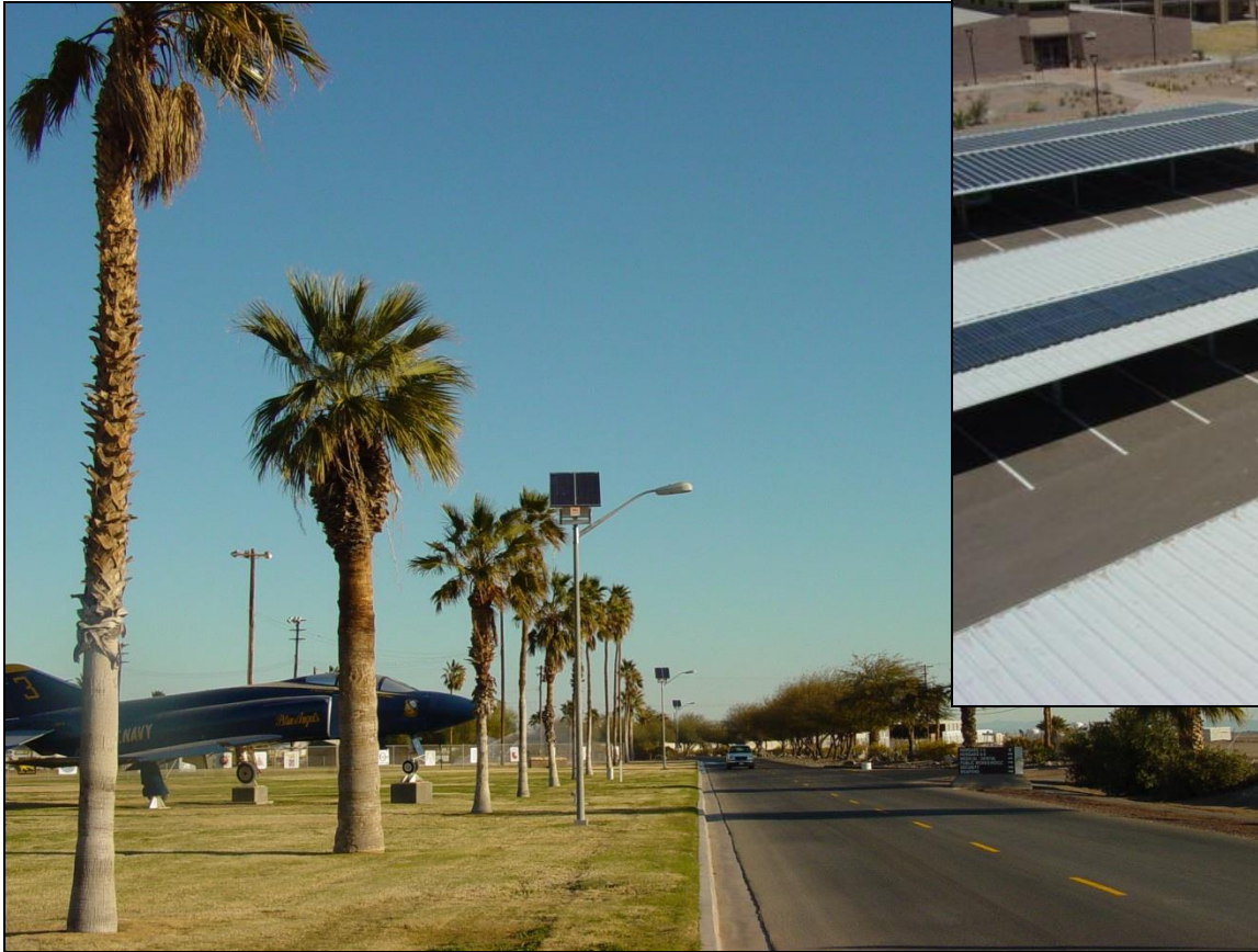
Solar Powered Streetlights
