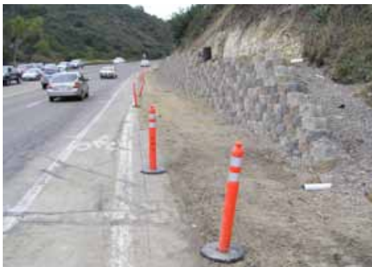
Texas Street Multi-Use Path under construction Photo: Andy Hamilton
