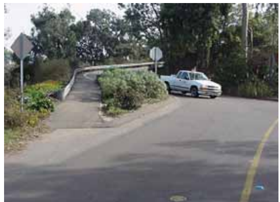
Curb extension and asphalt sidewalk, Del Mar
