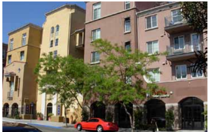
La Boheme, a mixed-use, infill project, 30th Street, San Diego Photo: Greg Konar
