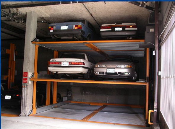
Triple-stack car-lift at the Berkeleyan, Berkeley, CA
